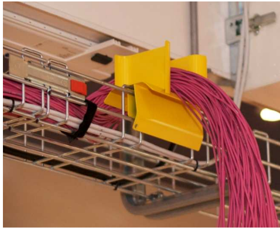
for Fiber cabling
